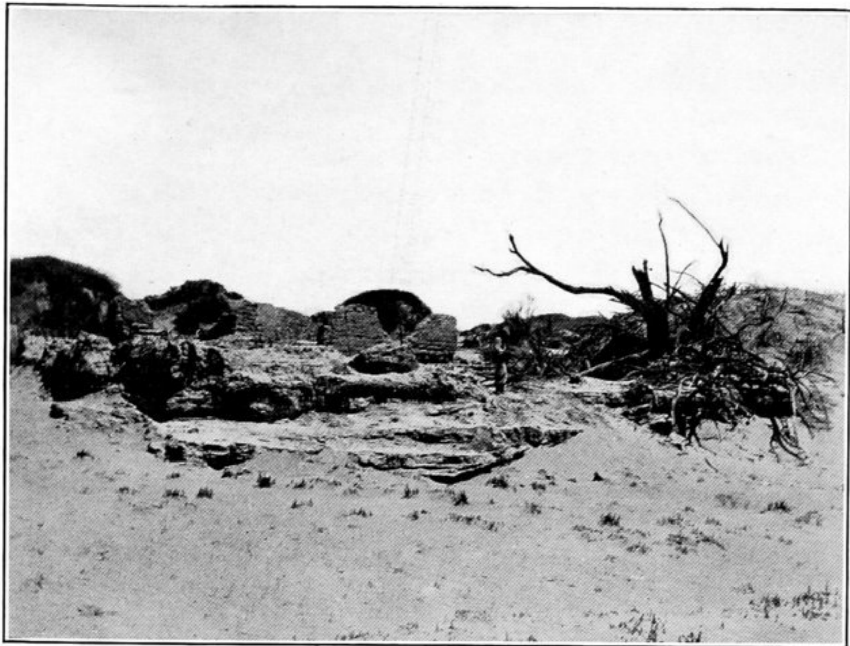
253. RUINED DWELLING, EAST OF K.K. IV, NEAR KHARA-KHOTO.
